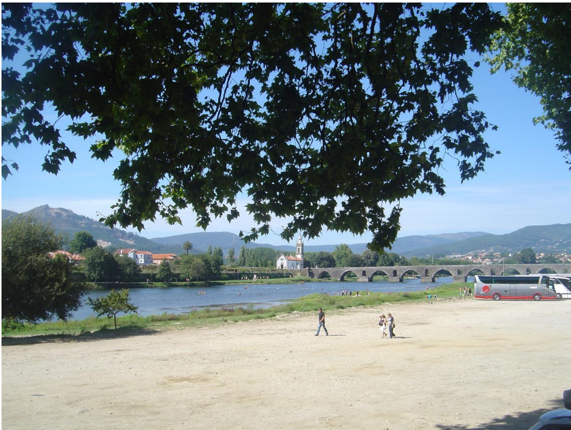
Fig. 2. Ponte de Lima bridge. Photograph by Ana Duarte Rodrigues.
