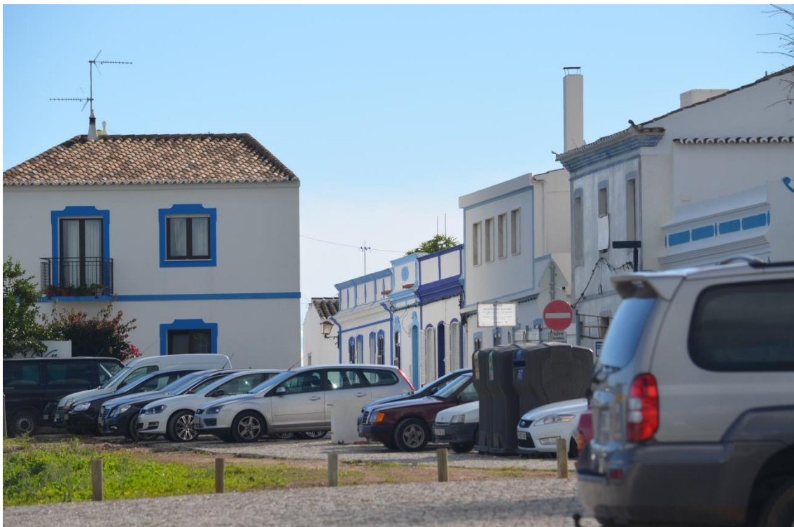
Fig.9. Adulteration of traditional architecture and car parking contributes to the degradation of the urban image. Photograph by Desidério Batista.
